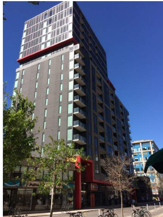
Existing 17-Storey Condominium Building at 435 Richmond Street West
