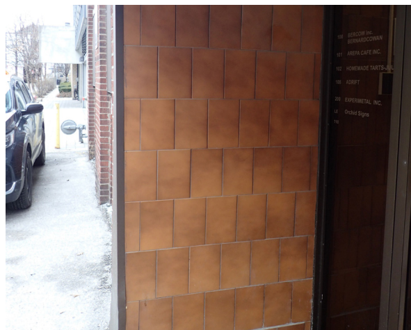
54. Fair condition of tiles at recessed entrance.
