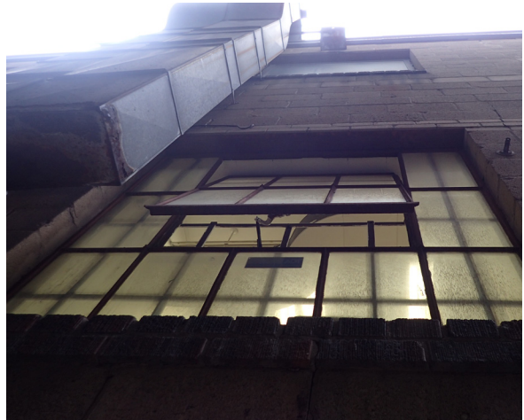
58. Operable steel window, West elevation.
