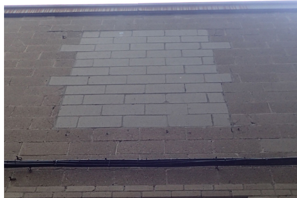
68. Infilled window, East elevation.
