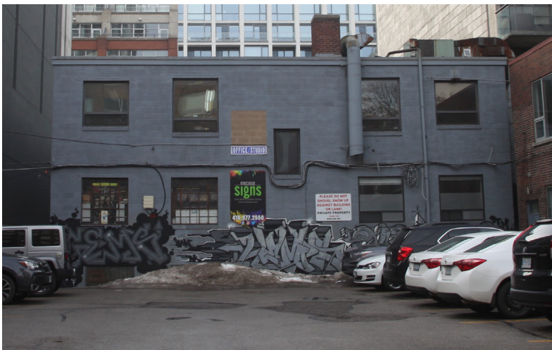
10. View of the rear (north) elevation of 38 Camden Street. (Source: ERA Architects).
