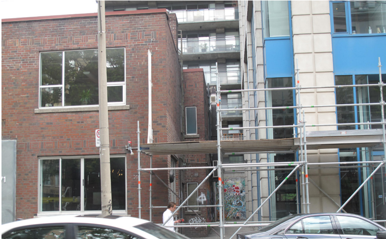
5. Partial view of 471 Richmond Street West's principal (north) and side (west) elevations. (Source: ERA Architects).
