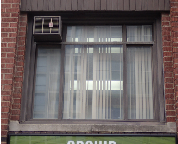
49. Fair condition of aluminium windows, South elevation.
