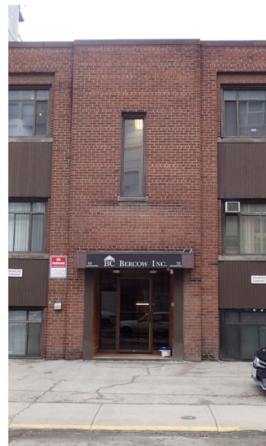
41. Central entrance to 38 Camden Street
