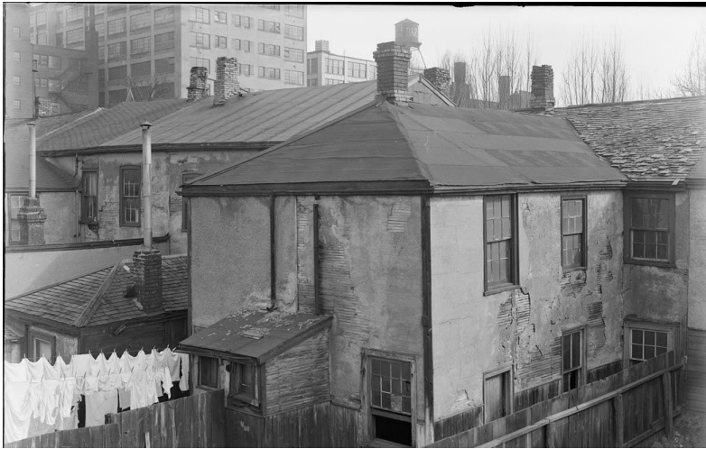
33. 1938 photograph of the rear of houses at 40-46 Camden Street, looking southeast. These houses would have been located immediately east of the Development Site, and reveal the poor condition of the area's first wave of residential development, as the neighbourhood transformed into an industrial hub. Large industrial warehouses on Spadina Avenue (including the Darling and Tower Buildings) can be seen in the background. (Source: City of Toronto Archives).
