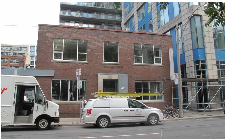
3. View of 471 Richmond Street West's principal (north) elevation. (Source: ERA Architects).
