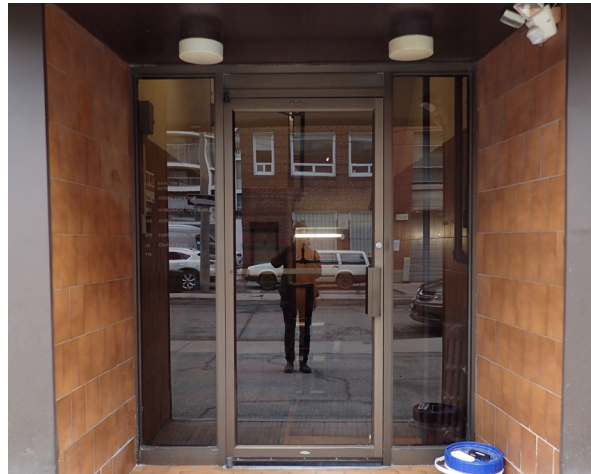
52. Fair condition of glazed aluminium entrance doors.
