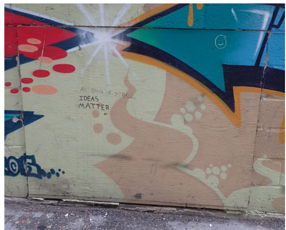
72. Protection board covering window opening, East elevation.
